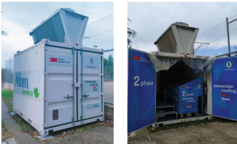
FIGURE 8 Two-phase immersion cooling EDC prototype.
